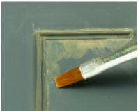
Use a flat brush moist with White Spirit and blend in the paint proximally 10 minutes after it is applied.
